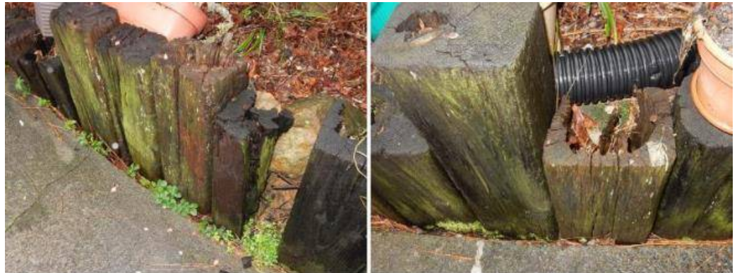
Water damage was noted in the crosstie retaining wall. It should be mentioned that most cross ties used for retaining walls and landscape timbers are 30 to 50 years of age. The decay noted in the cross ties should be monitored. Replacement will be needed. See photo
