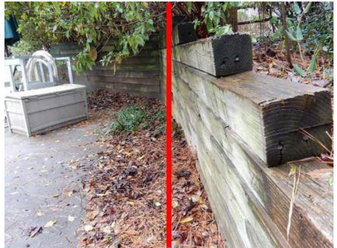
Water damage was noted in the crosstie retaining wall. It should be mentioned that most cross ties used for retaining walls and landscape timbers are 30 to 50 years of age. The decay noted in the cross ties should be monitored. Replacement will be needed. See photo
