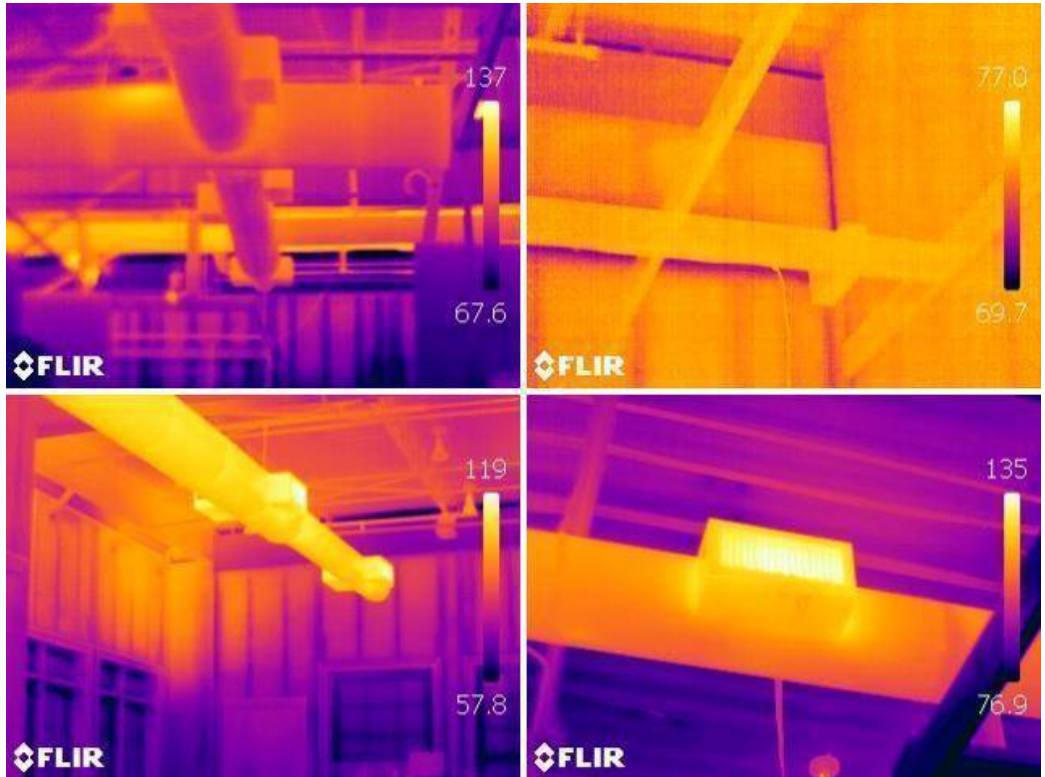
Infrared Scanning of air ducts and roof decking for leaks.
